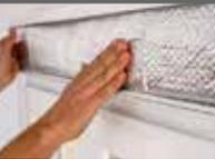
Isolate the windows and window shutters with thermal isolation materials.
